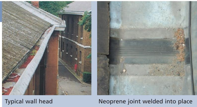
Fig 2. Flexible Expansion Joint
